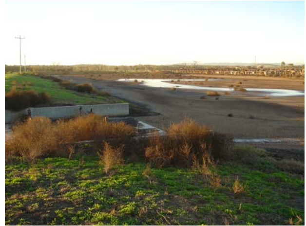
Debris Basin, typical outlet structure used on AU feedlots is a flume or porous dam outlet structure.
