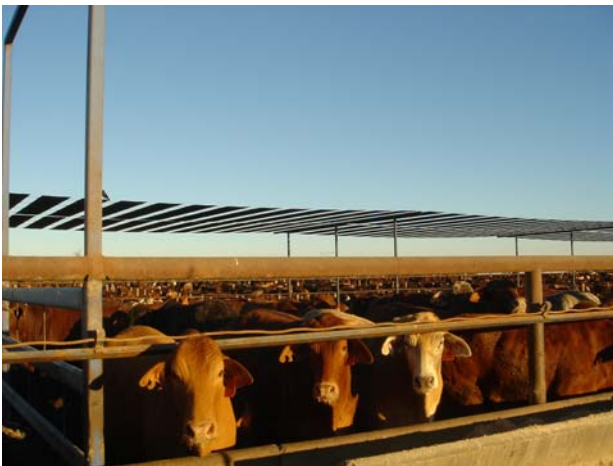
Shade structures, a different structure than typically seen, they are sheets of tin, instead of shadecloth, less susceptible to wind damage.
